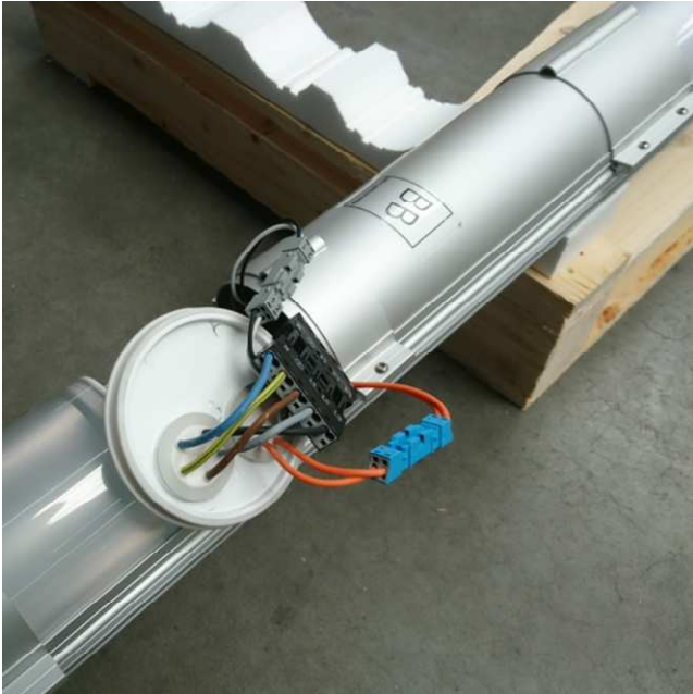
Picture 1: Connect the Plug & play connectors
